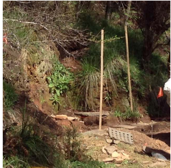
Above - Part of the excavation site.
